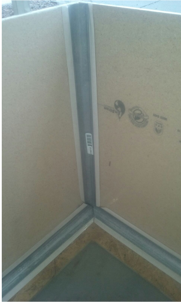
Figure 5: This figure shows the three-way intersection. It will come out of the mold rough, and it will be sanded to a smooth round corner.
